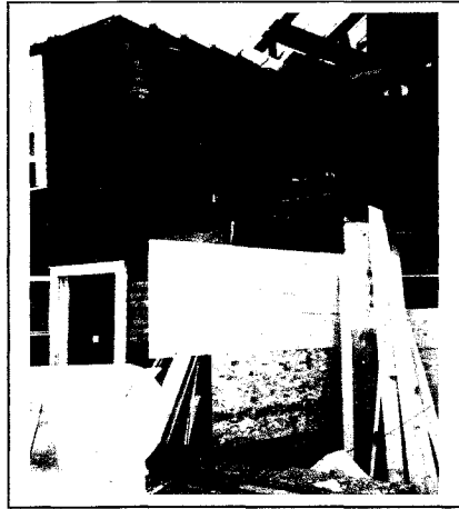
Figure 8: Condition of Bob’s project house after removal of an inappropriate addition.
